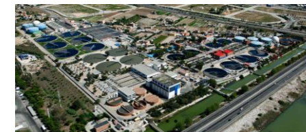
WWTP Pinedo Valencia (Spain)
