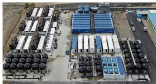
Hsinchu Emergency Desalination Plant — 13,000 tons/day Output
