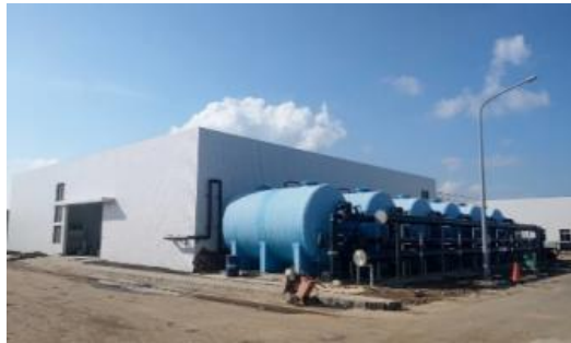
Hsinchu Desalination Plant
