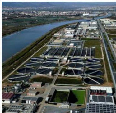
A&WWTP Depur-Baix (BCN) Spain Multipurpose WRP - IPR
